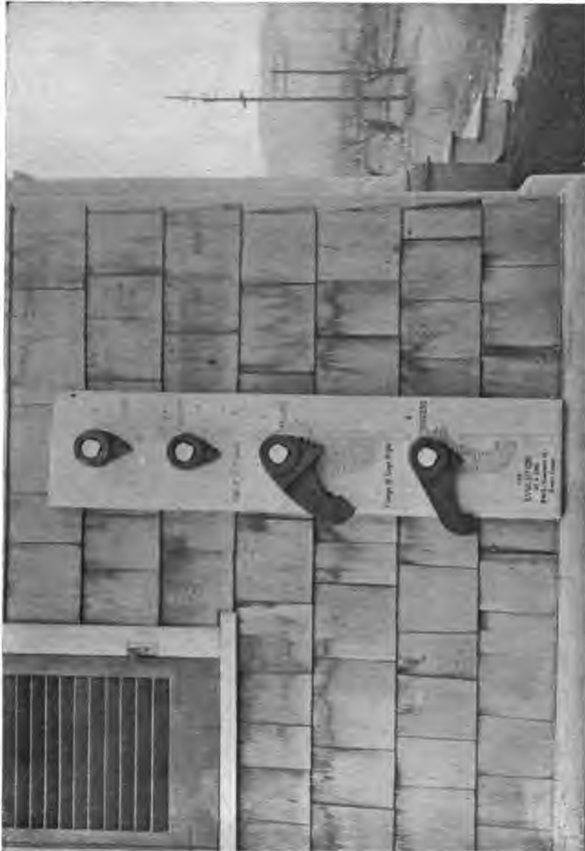
PLATE 85.—Contract 12. Various Types of Safety Dogs Used on Cages Operating in Shafts of Rondout Siphon. Lowest dog was found to be satisfactory.
